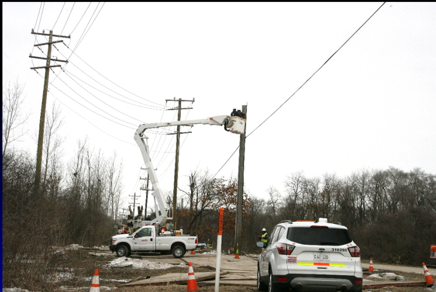
Com Ed and Nicor gas crews relocate power poles and lines while Homer Tree removes trees and brush along IL 25 for the LMP Section C-3 IL 25 Intersection Improvement project
