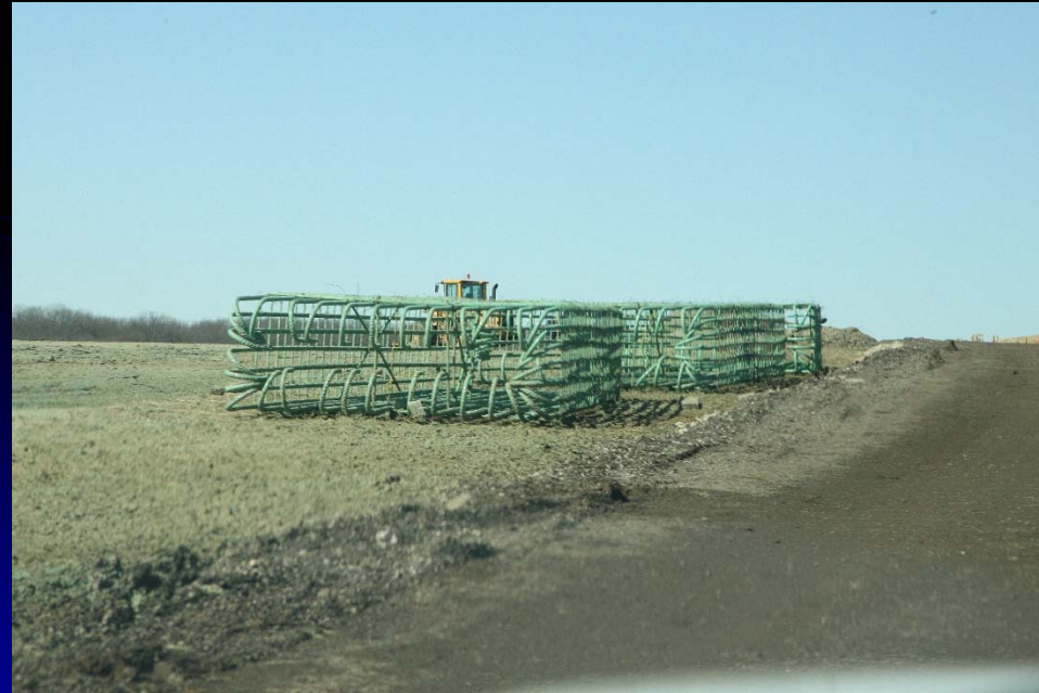
Crews work on driving foundation piles and fabricating pier reinforcement cages for the LMP C1- East of IL 31 to Sandbloom Road project
