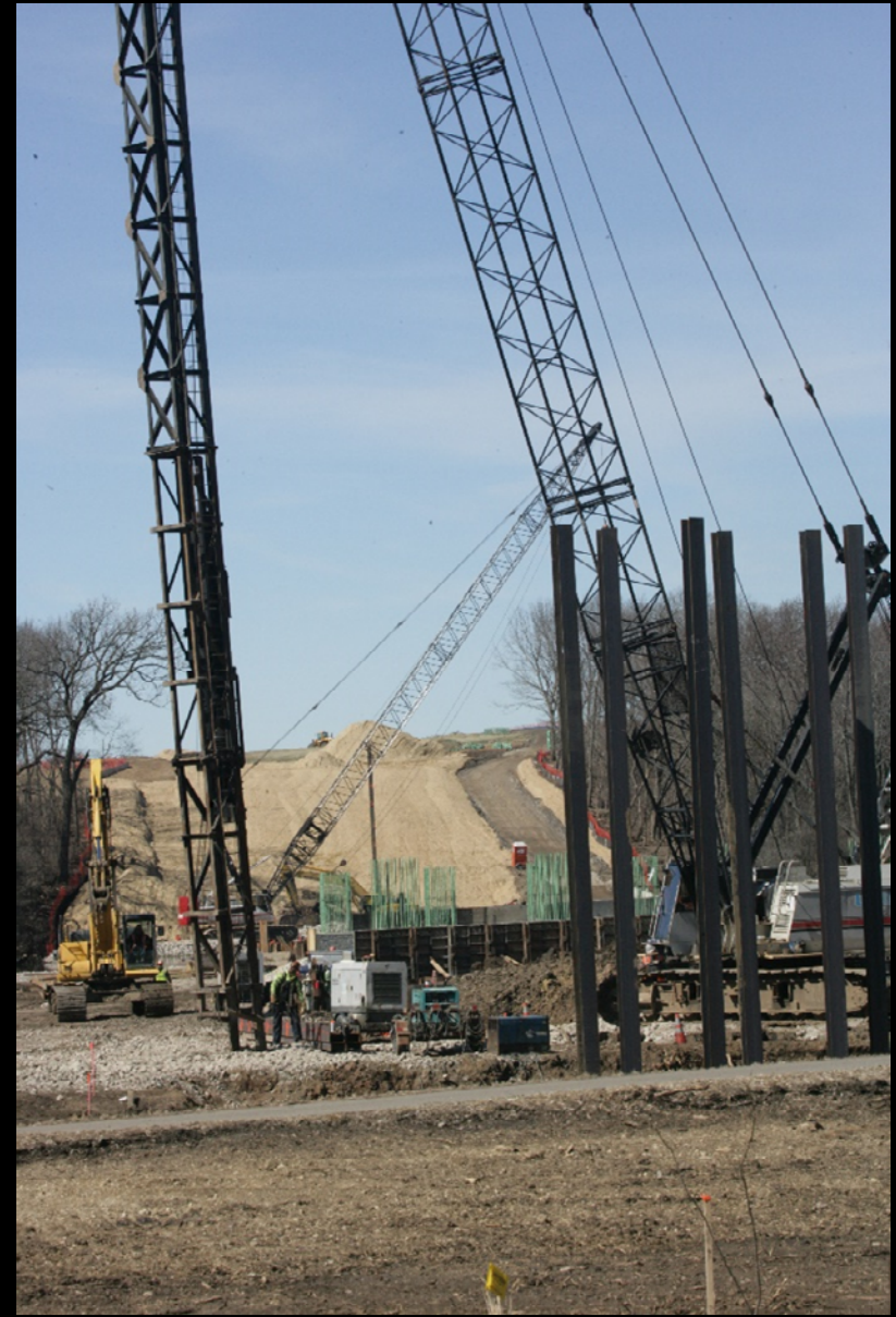
Crews work on driving foundation piles and fabricating pier reinforcement cages for the LMP C1- East of IL 31 to Sandbloom Road project
