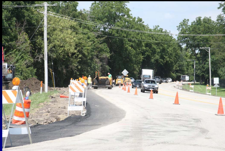
Crews widen pavement and work on electrical features for the Kirk Road at Dunham Road Intersection Improvement project
