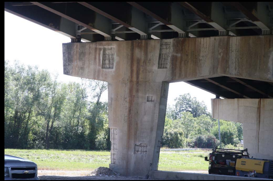
Crews work on pier concrete repairs on the Structural Bridge Rehab #1 project.
