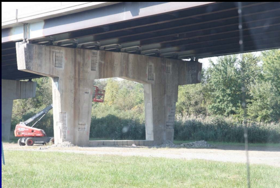
Crews work on pier concrete repairs on the Structural Bridge Rehab #1 project.
