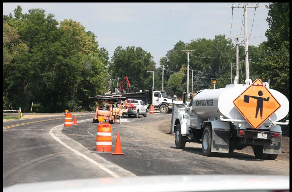
Crews widen pavement and work on electrical features for the Kirk Road at Dunham Road Intersection Improvement project
